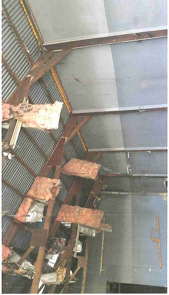
Fig. 6 - Interior Frame East Side of South End Room
